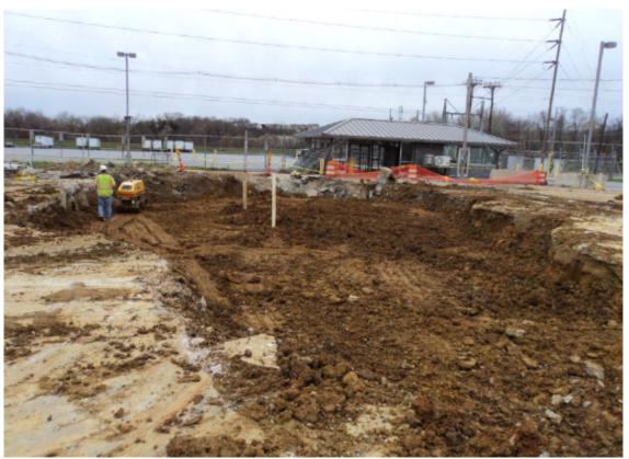
A45: View (looking west) of partially backfilled excavation and infiltration gallery (PVC uprights) at the northwest corner of former Building 4.
