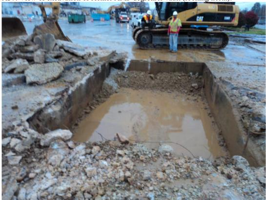
A38: View of excavation of former AMF degreaser vault (looking south). Dimensions are approximately 12' (E-W) by 20' (N-S), and 3' deep.
