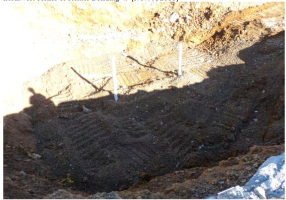
A44: View (looking northeast) of infiltration gallery installation in excavation at the northwest corner of former Bldg 4. [Nov. 9, 2011]. Stone backfilled to approx. 16' bgs.
