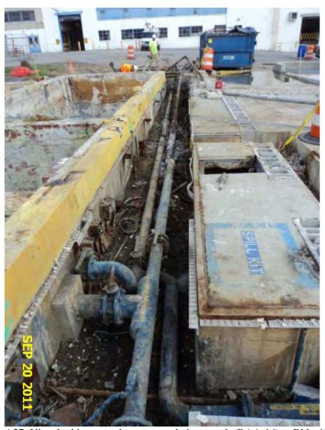
A27: View looking east along exposed pipe trench (RAA-16) at Bldg 41 (Bldg 42 in background). Photo is after building demolition and prior to pipe removal and remediation.
