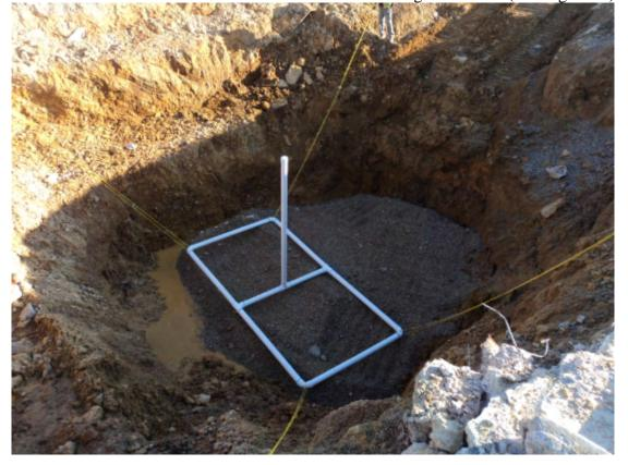
A41: View (looking northeast) of infiltration gallery installation in excavation at the northwest corner of former Building 4. [Nov. 9, 2011] Note gravel layer (approx 2' thick) placed beneath gallery.
