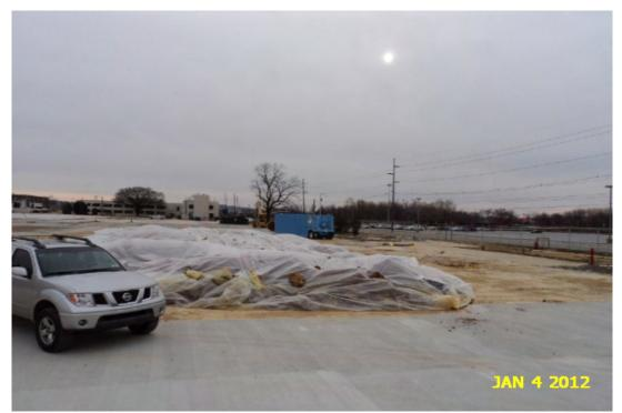
A51: View looking south from north end of former Bldg 4 – of stockpiled hazardous soil and blue frac tank with hazardous remediation liquid.
