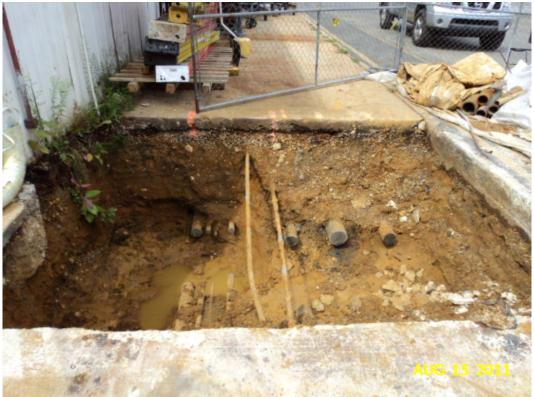
A13: Photo of one pipe cleaning excavation following cleaning and capping of pipe [prior to backfill].
