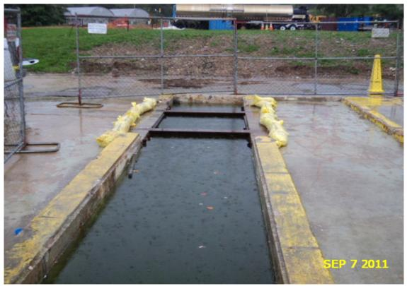
A26: View looking north of former sludge pit filling with rainwater following demolition of building 41 above-ground structure. Note sand bags lined on ground in attempts to slow run-in.
