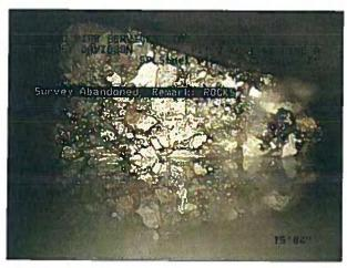
Photo: 24\_2a, Tape/Media No.: HD-1, 01:09:37 15.3FT, Obstacles Rocks, 100 % of cross sectional area, from 12 to 12 o'clock
