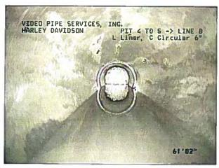
Photo: 43\_3a, Tape/Media No.: HD-1, 01:34:38 61.2FT, End of Pipe, Remark: CAPPED
