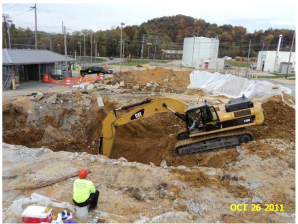
A34: View (looking north) of soil removal surrounding the former below grade degreaser vault at the north west corner of former Building 4. Note Gate 4 and north fire protection pump house in background.
