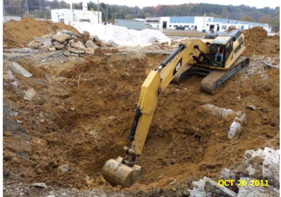
A33: View (looking northeast) of soil removal surrounding the former below grade degreaser vault at the north west corner of former Bldg 4. Note remnant of former southeast corner base of vault below trackhoe. Total depth at bottom is approx. 23' bgs.
