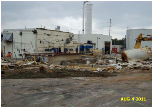
A24: View looking west at Building 41 (wastewater treatment building) during demolition. Note EQ tank and green marks on asphalt (fmr underground ww piping).
