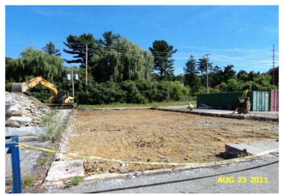
A16: View looking north at Bldg 51 following demolition and removal of former hazardous waste storage pad and underlying gravel, and prior to confirmation sampling.
