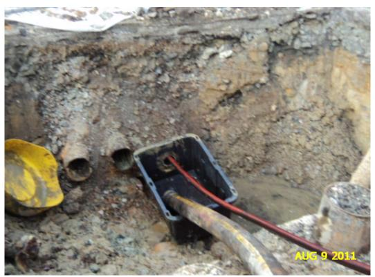
A12: Photo of underground pipe cleaning technique – high pressure wash while vacuum removal and onsite containment.
