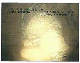
Photo: 36\_3a, Tape/Media No.: HD-1, 01:24:21 26.8FT, Collapse Pipe Sewer, 100 %
