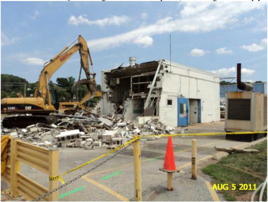
A25: View looking northeast at Bldg 41 during demo. Note green markings on asphalt showing the location of former underground cyanide wastewater piping (from Bldg 4).
