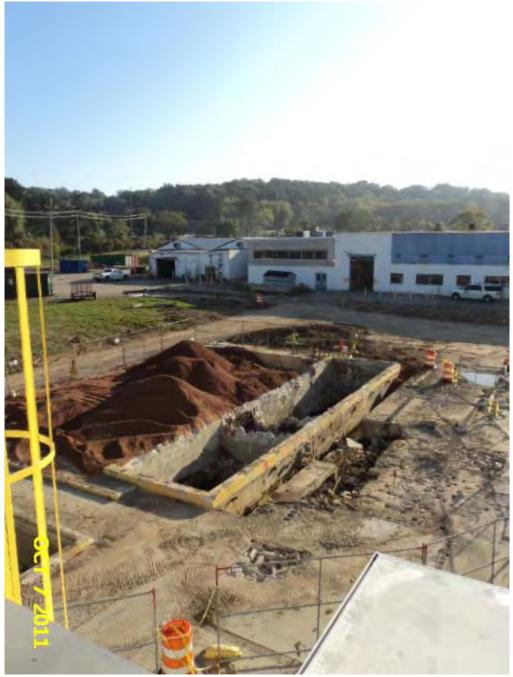
A30: View looking northeast of partial remediation and backfill of the former wastewater treatment facility at Building 41 (Building 42/57 is in the background).
